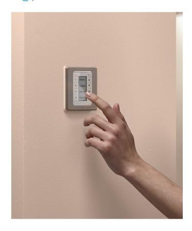
The new E-ink scene plate from CP Electronics allows for the control of complex lighting scenes as part of the An-10 lighting control system.
